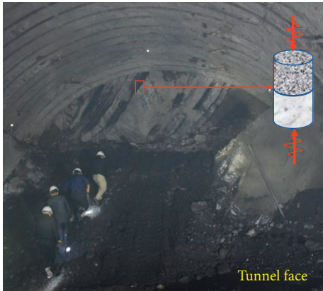
FIGURE 1: Photograph of composite rock in tunnel face.
