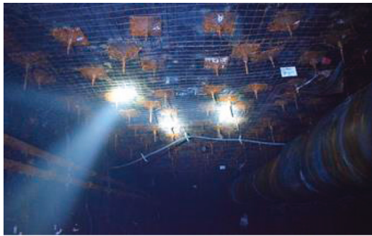
FIGURE 13: Photos of Roadway maintenance effect.
