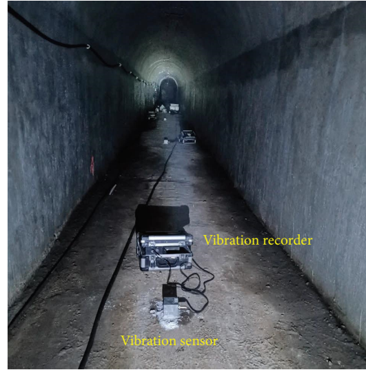
FIGURE 3: Blasting vibration monitoring.
