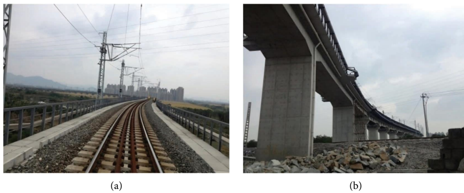
FIGURE 4: Railway line and bridge appearance. (a) Railway line. (b) Bridge.
