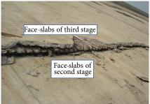
(b) Dislocations after cleaning up the damaged concrete
