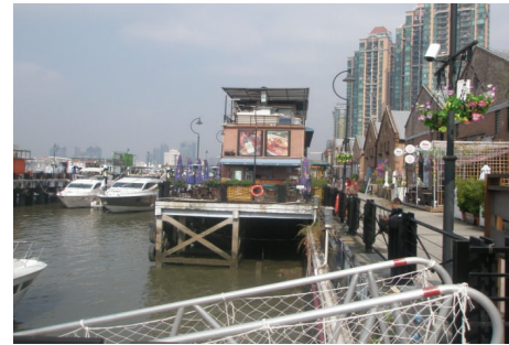
FIGURE 5: Riverside view of Taikoo Wharf.
