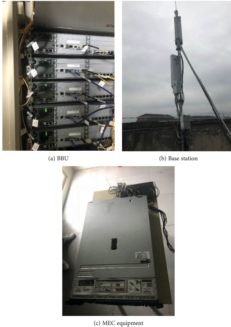
FIGURE 8: Part of the equipment used in the test.
