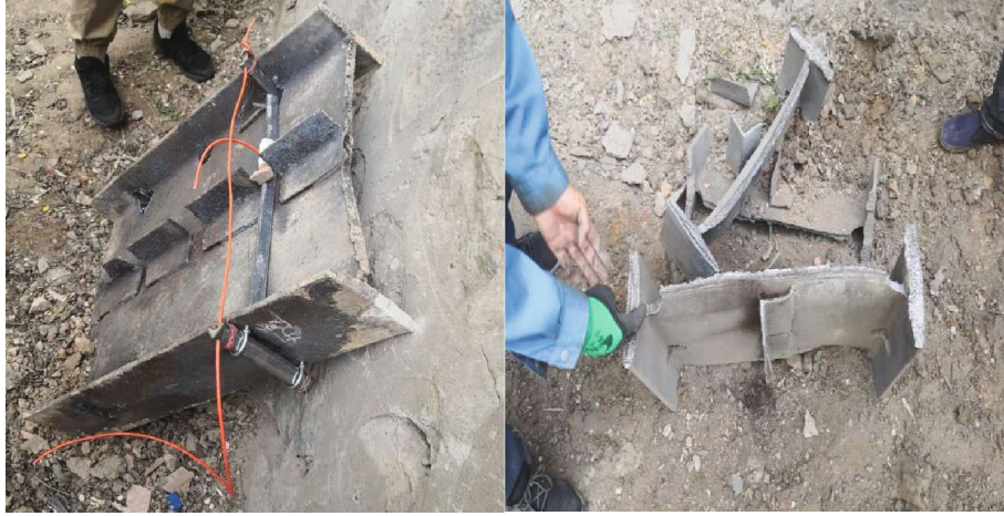
FIGURE 6: Before and after cutting the vertical support I -beam.
