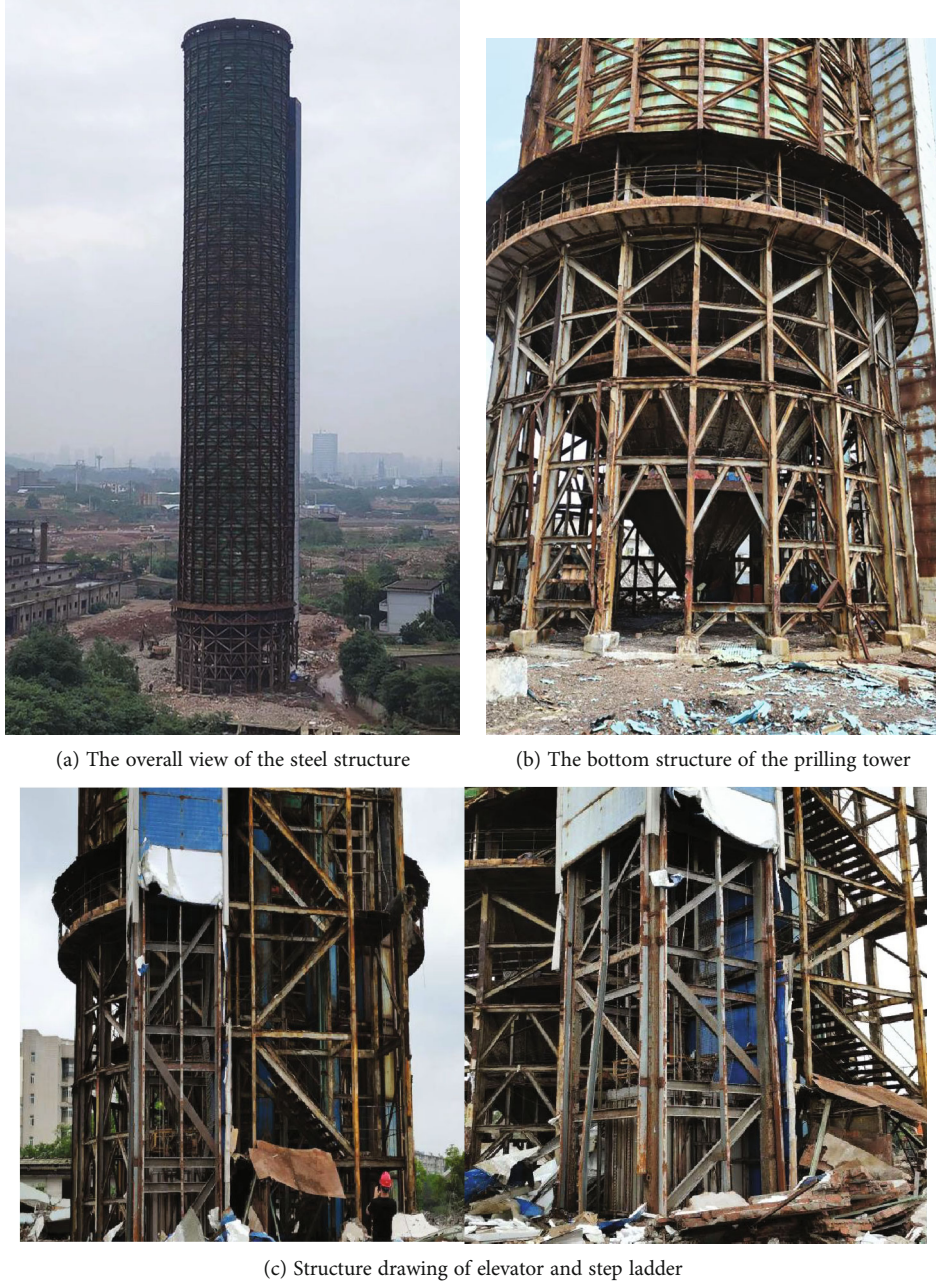
FIGURE 2: Structural drawing of steel structure.
