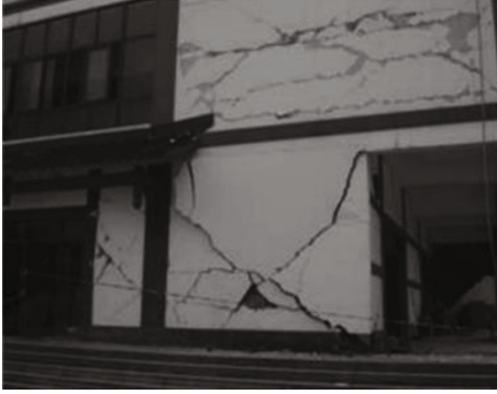
FIGURE 1: X-shaped crack.
